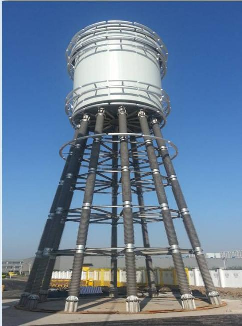
**4. Smoothing reactor:** A *smoothing reactor* is connected in series with the DC high voltage line as either part of the converter station or back to back interconnection between different transmission networks. It reduces the harmonic current [ripple], limits the inrush current during fault conditions, limits the DC phase current rate of rise and improves the dynamic stability of the power system.
