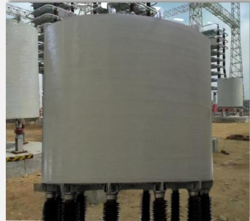
**3. Current-limiting reactor:** A current limiting reactor is connected in series with the power system. It is designed to reduce short-circuit currents, which result from plant expansions and power source additions, to levels that can be adequately handled by existing transmission and distribution equipment.
