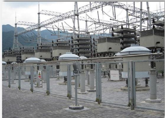
**6. Damping reactor:** A damping reactor is connected in series with one or more capacitor banks. It is designed to limit the capacitor switching inrush current while also capable to withstand the rated current and fault current in the event of a short circuit.
