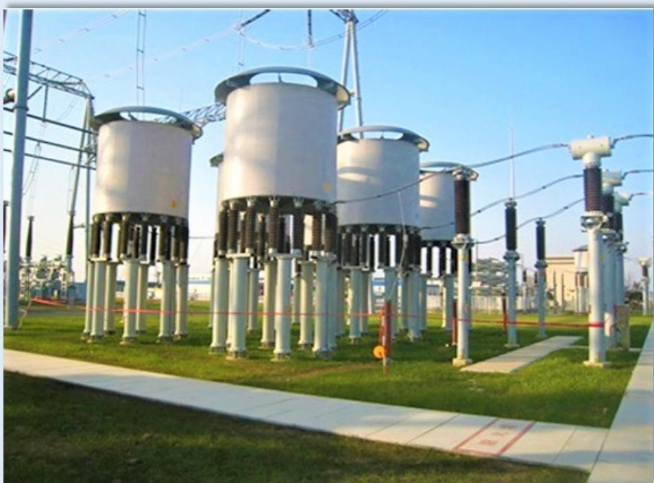
**2. Thyristor controlled reactor:** A thyristor-controlled reactor [TCR] is a reactor connected in series with a bidirectional thyristor valve. The thyristor valve is phase controlled, which allows the value of delivered reactive power to be adjusted to meet varying system conditions.
