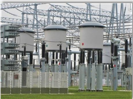
**7. Test reactor:** Test reactors are installed in high-voltage and high-power laboratories. The typical applications include: current limiting, synthetic testing of circuit-breakers, inductive energy storage, and simulation circuits.
